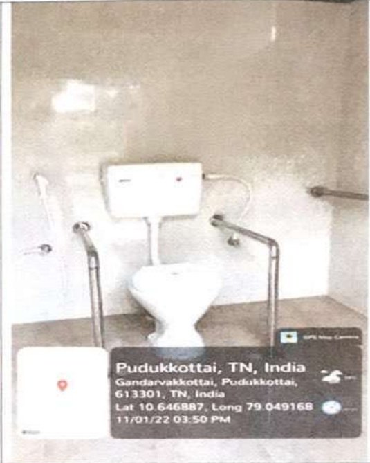
Divyangjan Toilet view II
