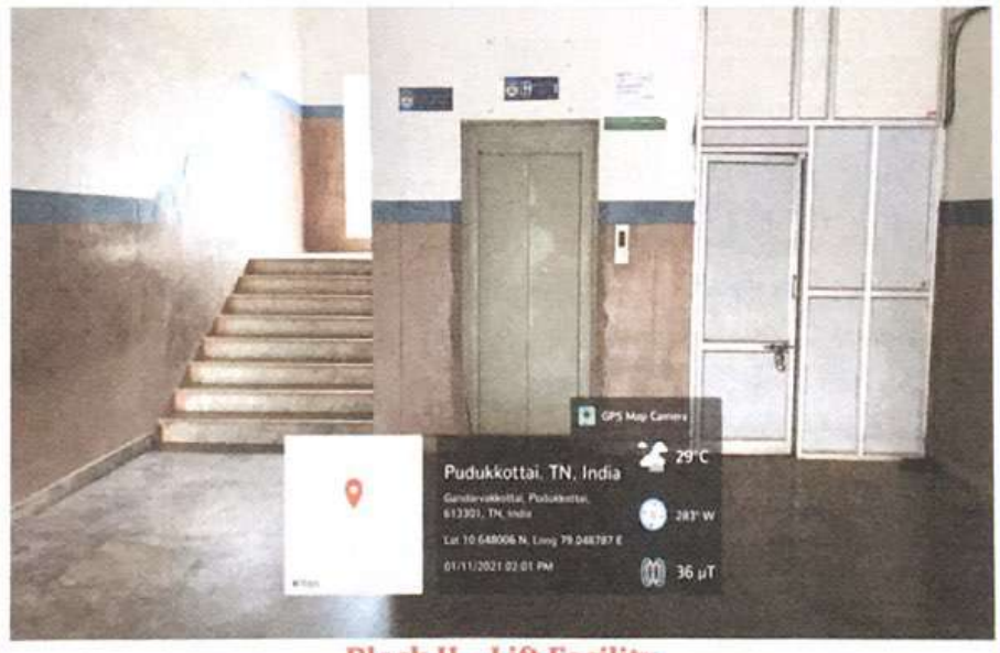
Block II - Lift Facility
