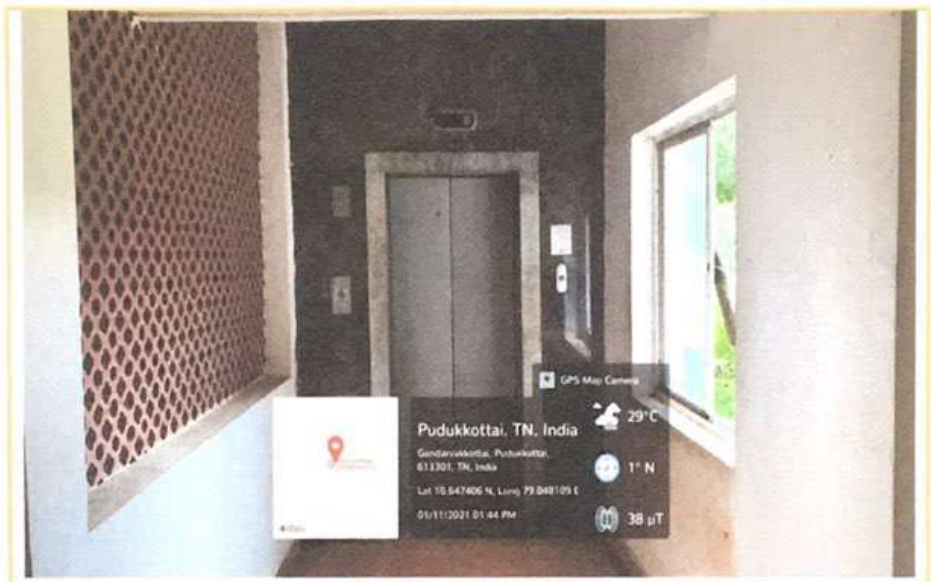
Block I - Lift Facility
