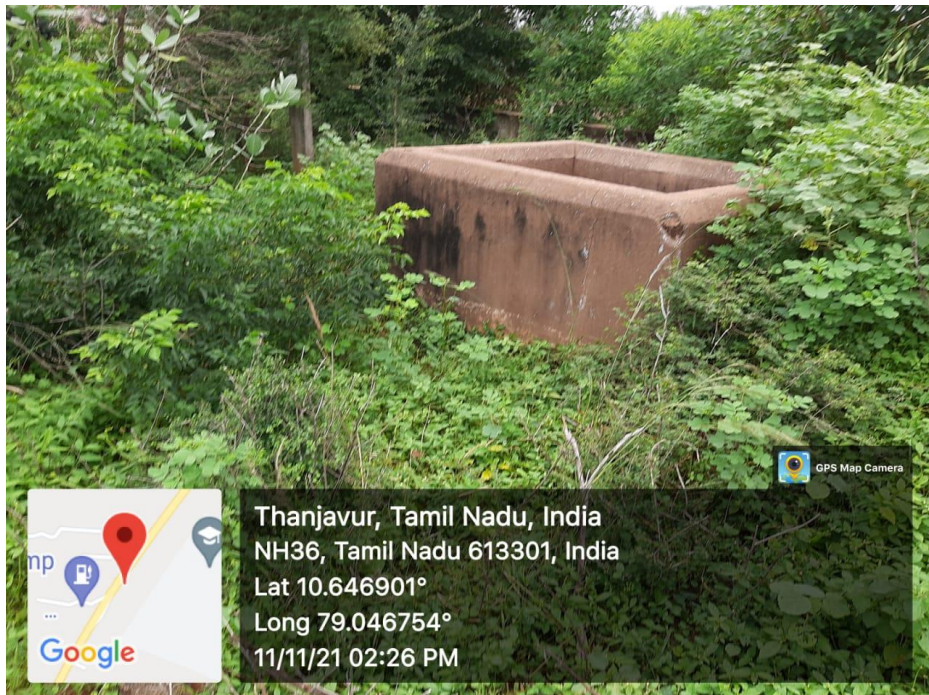
Degradable and non- degradable waste storage
